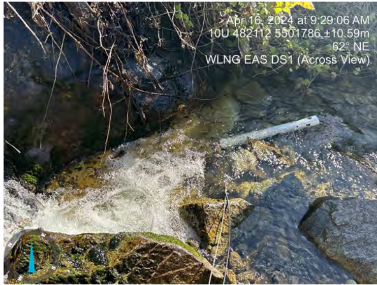
Photo: 3 Location: EAS DS1 Description: Across View
