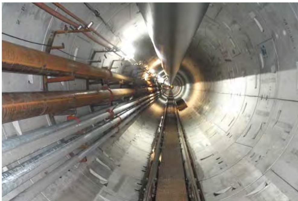
Figure 2. Fully-assembled Precast Concrete Segmental Tunnel Liner Installed as the TBM Advanced
