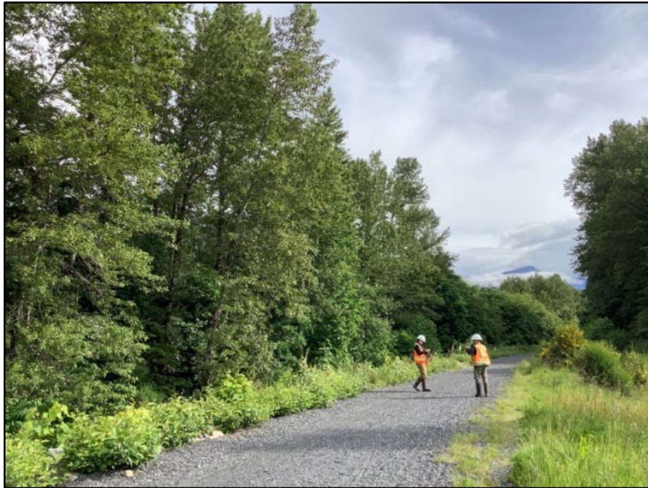
Photo 1. View north along the dike, east of the existing discharge outfall. The outfall is located on the left, on the far side of the riparian community (June 10, 2021).
