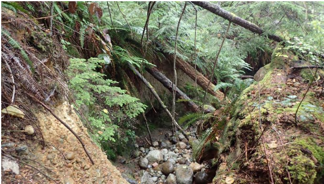
Figure 2 Scouring and Erosion along Reach B Stream X, August 20, 2020
