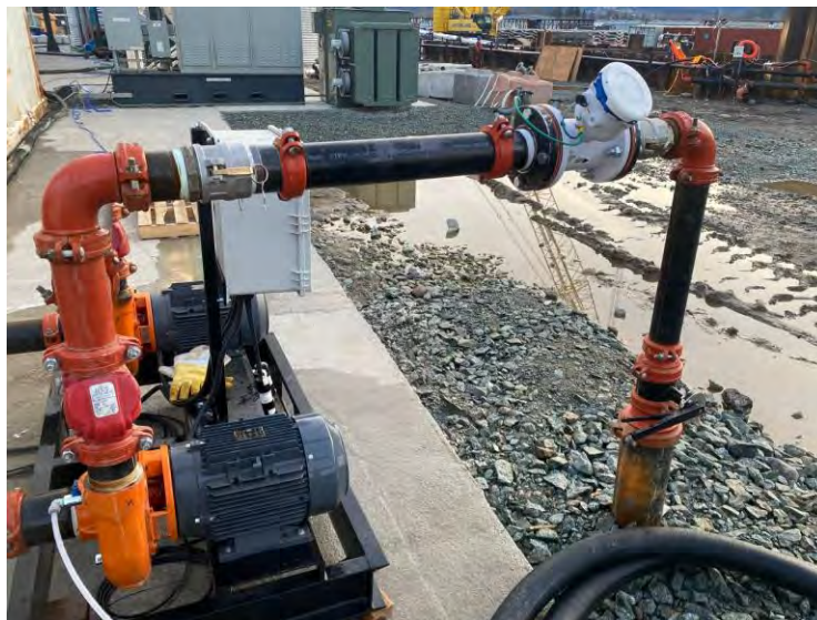
Photo 8: 04:53 PM, 03/15/24 (Flow Meter installed on the discharging pipe)
