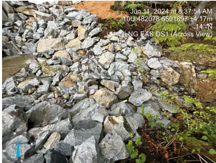
Photo: 2 Location: EAS DS 1 Description: Across view
