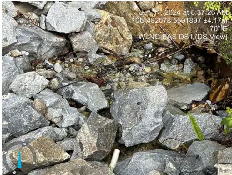
Photo: 3 Location: EAS DS 1 Description: DS view
