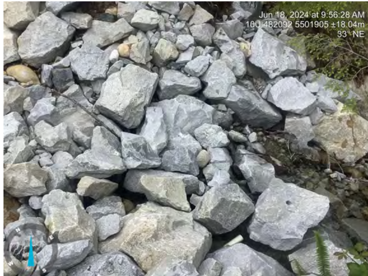
Photo: 2 Location: WLNG DS 1 Description: Across view
