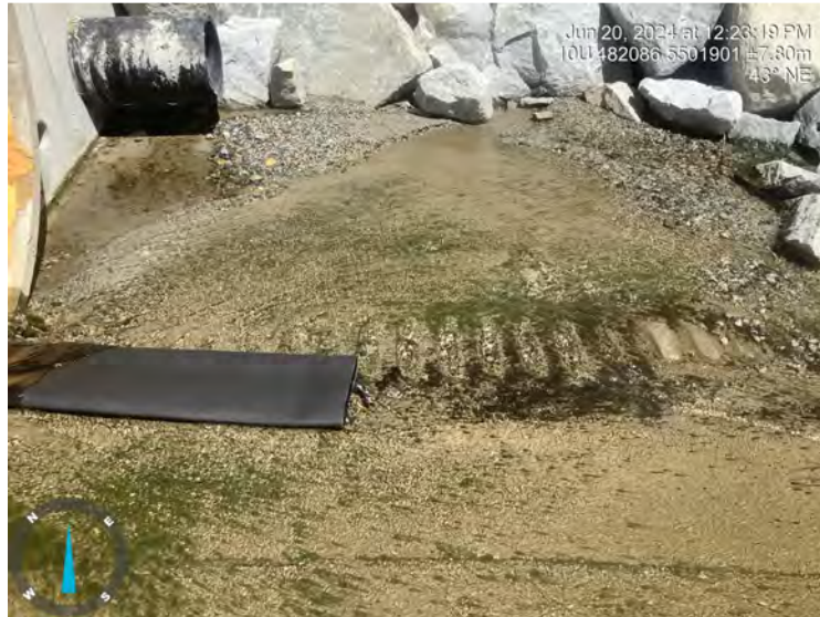
Photo: 2 Location: WLNG EOP Across View Description: WLNG EOP Across View
