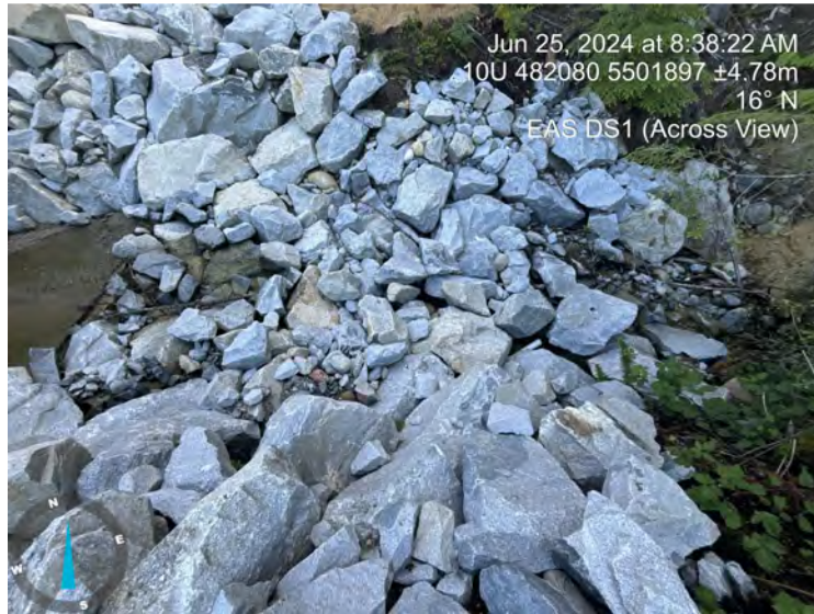
Photo: 3 Location: EAS DS1 Description: Across View
