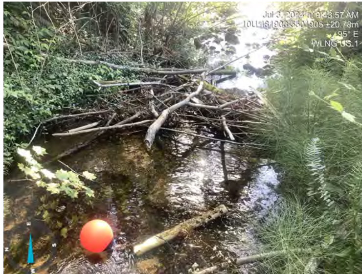
Photo: 3 Location: EAS US 1 Description: DS view
