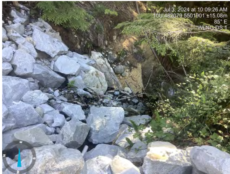
Photo: 3 Location: EAS DS 1 Description: DS view
