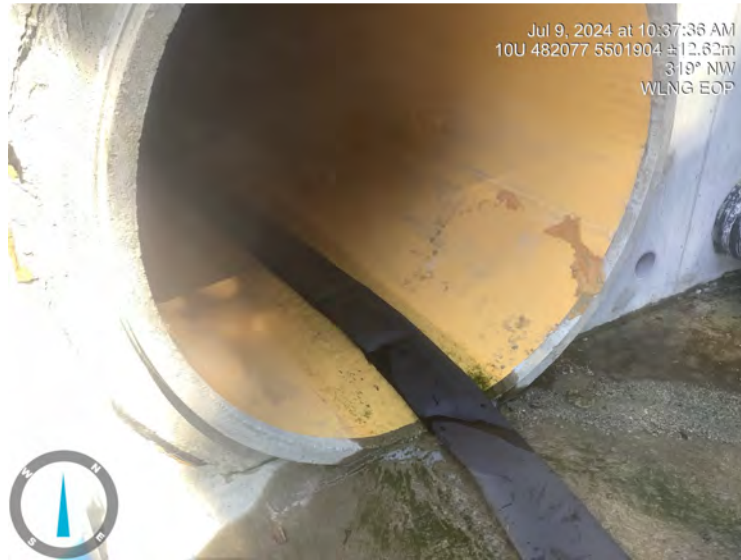
Photo: 1 Location: WLNG EOP Description: US view
