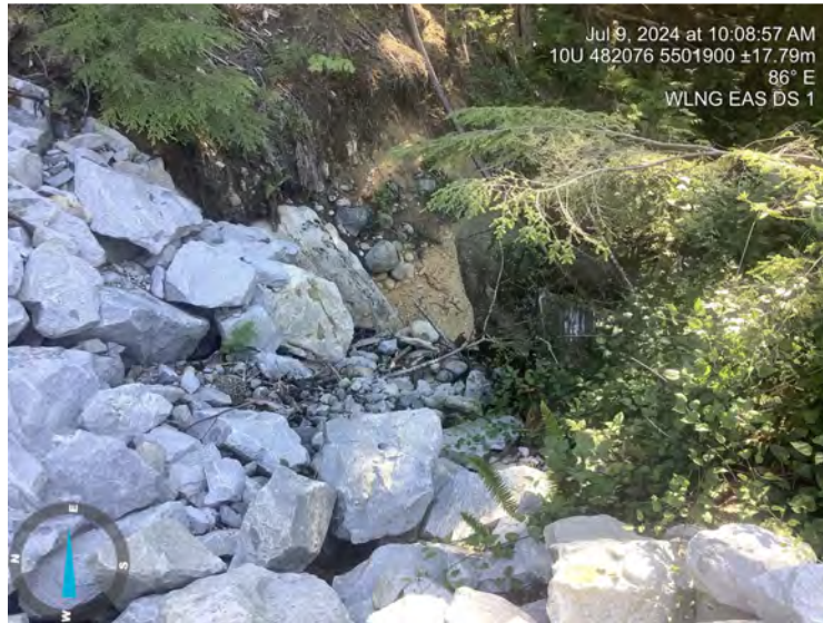
Photo: 3 Location: EAS DS 1 Description: DS view
