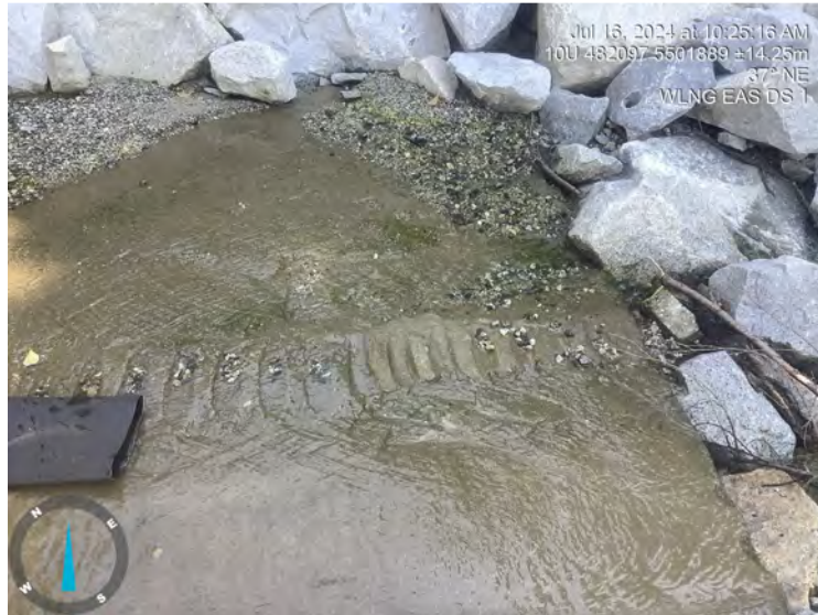
Photo: 2 Location: EAS DS 1 Description: Across view
