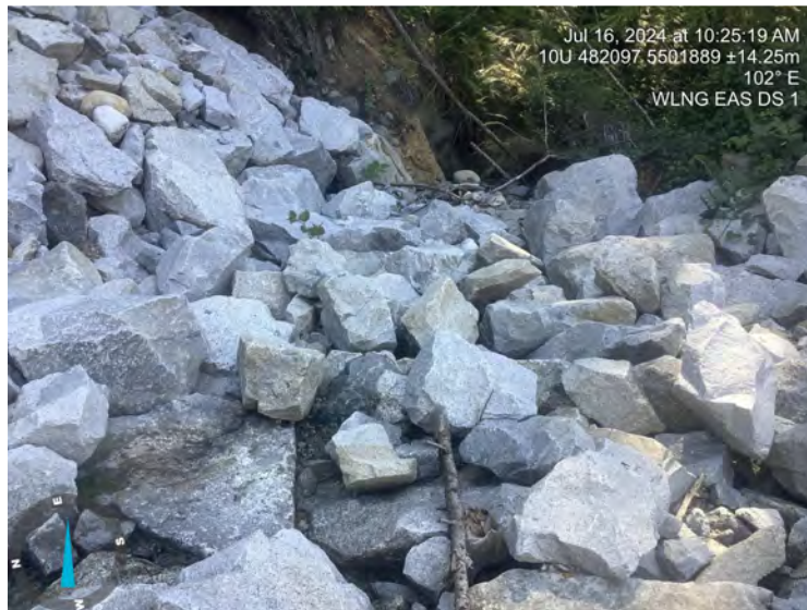
Photo: 3 Location: EAS DS 1 Description: DS view
