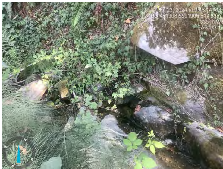
Photo: 1 Location: EAS US 1 Description: US view
