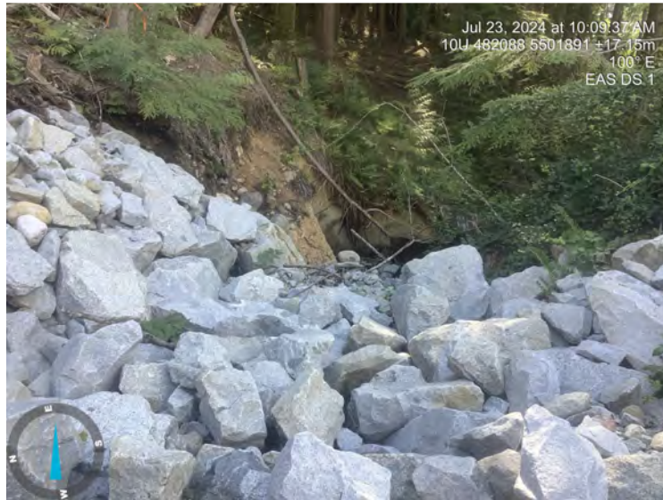
Photo: 3 Location: EAS DS 1 Description: DS view
