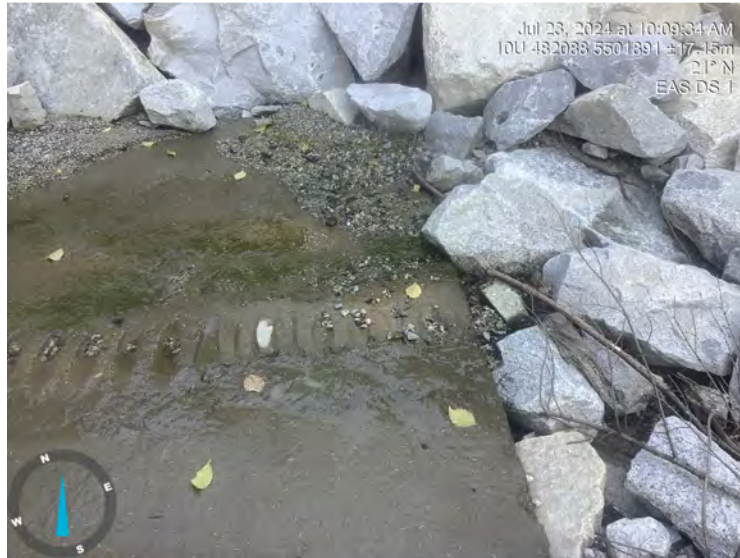
Photo: 2 Location: EAS DS 1 Description: Across view
