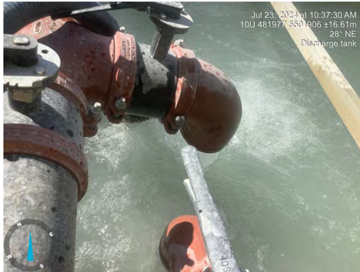
Photo: 1 Location: W LNG EOP tank Description: View into tank
