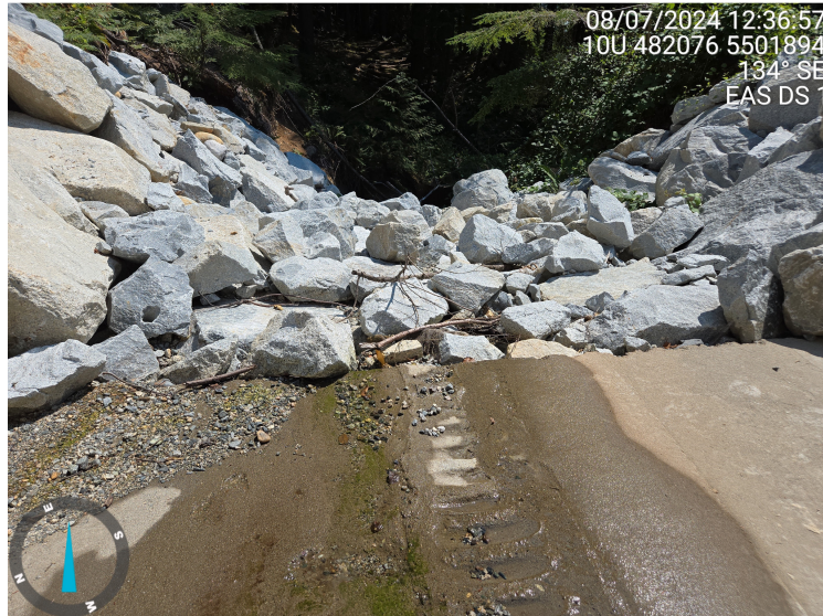
Photo: 2 Location: EAS DS 1 - original Description: Low flow DS view
