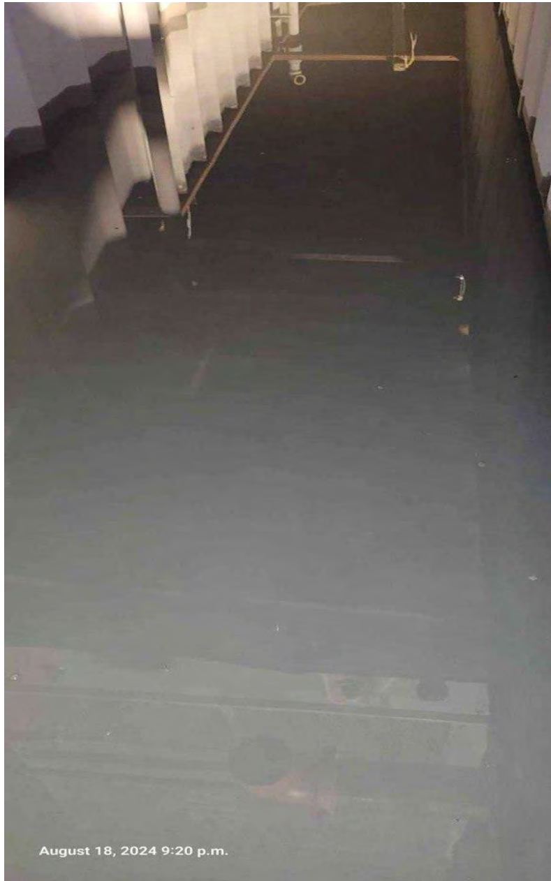
Photo 17: Top of the WTP tank 08/18/2024
