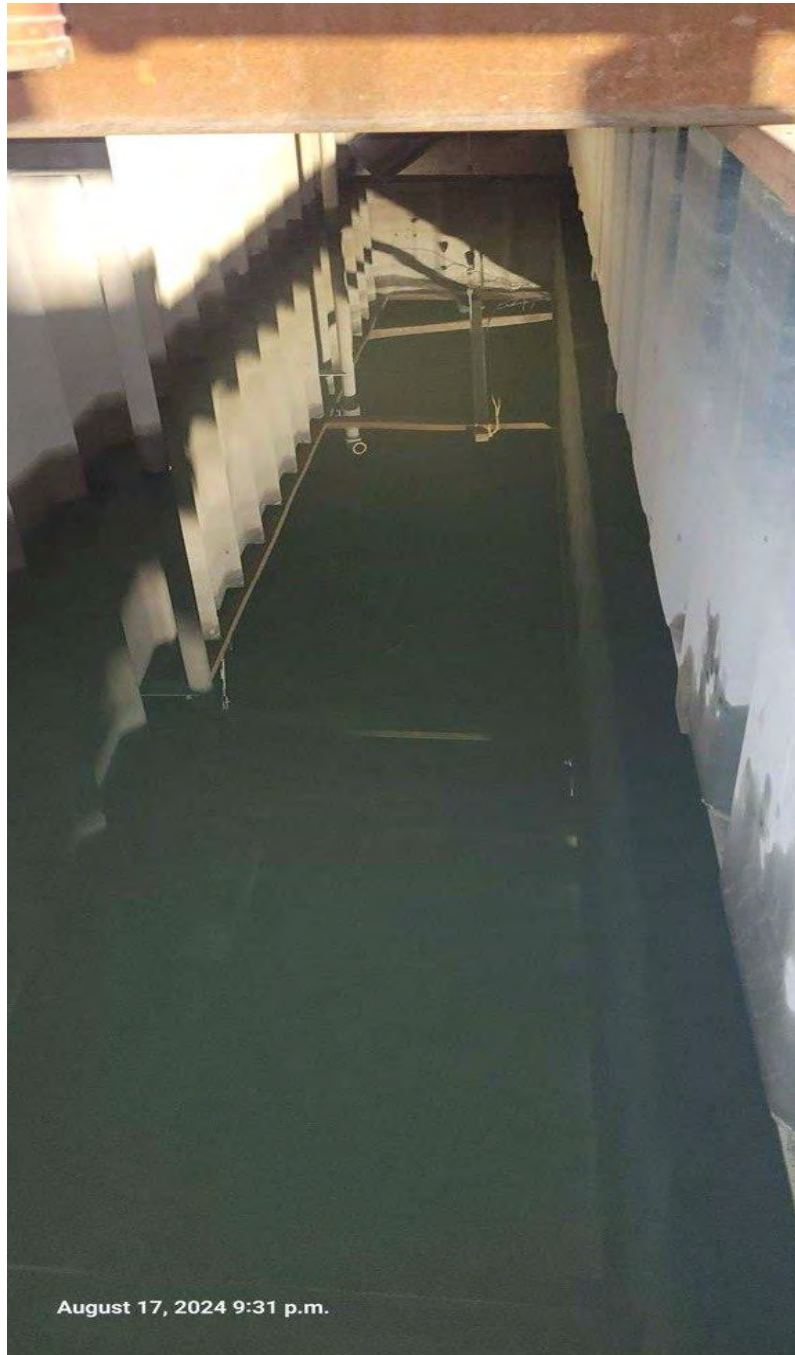
Photo 13: Top of the WTP tank 08/17/2024
