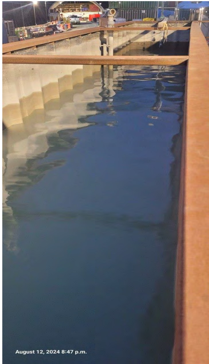
Photo 2: Top of the WTP tank 08/12/2024
