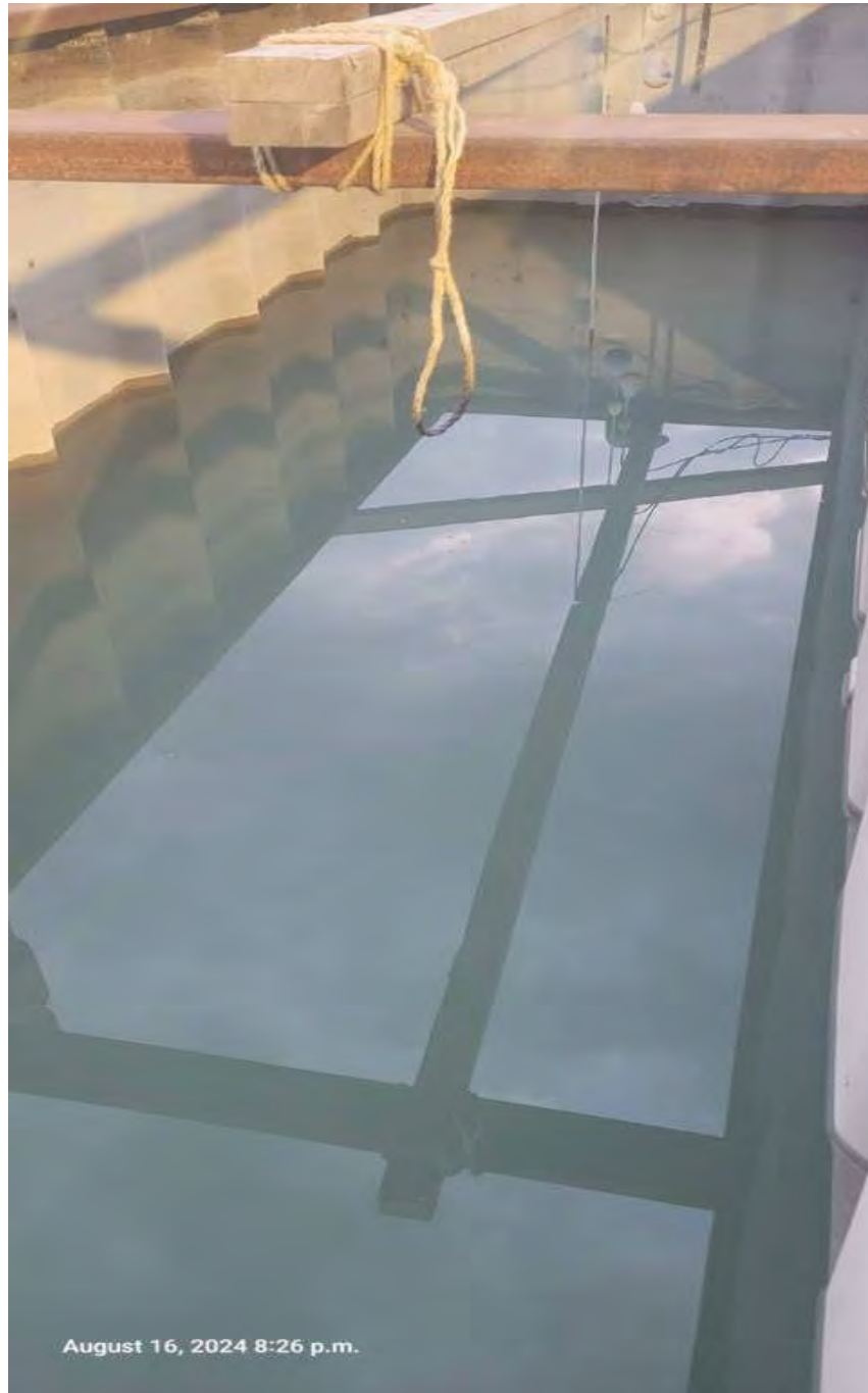
Photo 11: Top of the WTP tank 08/16/2024
