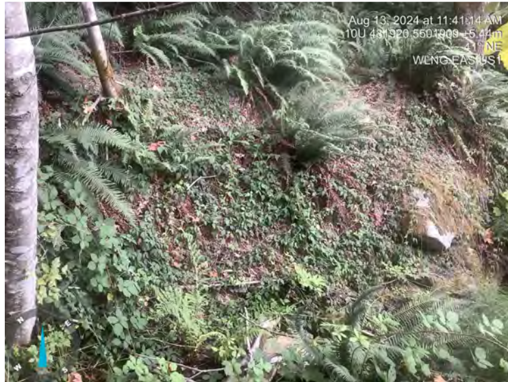
Photo: 2 Location: WLNG EAS US1 Description: Across view
