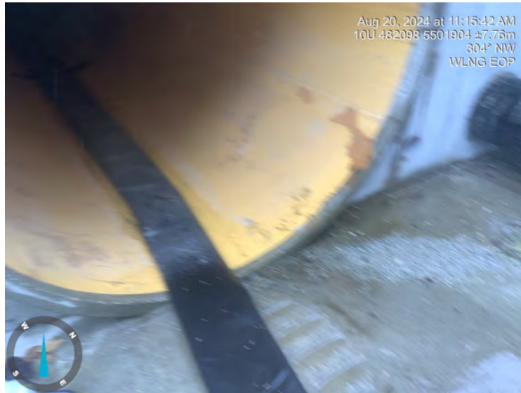
Photo: 1 Location: WLNG EOP Description: US view
