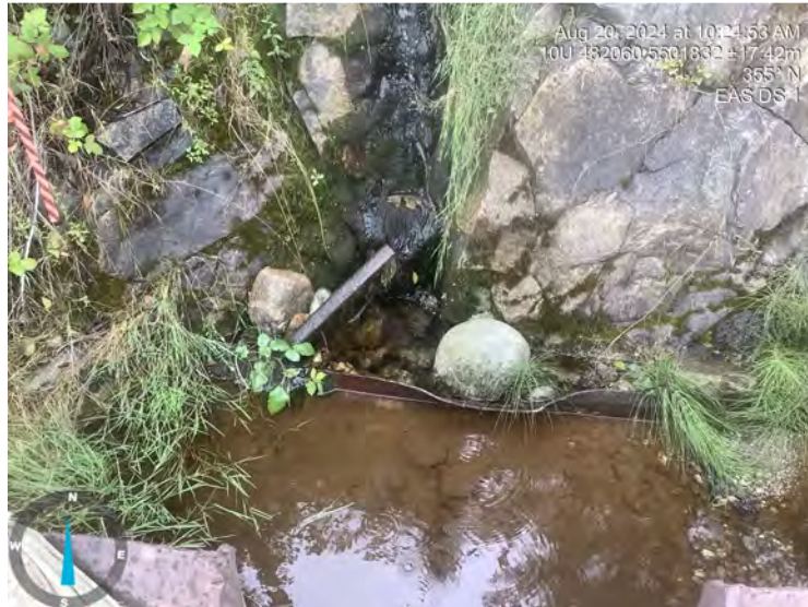
Photo: 2 Location: EAS DS 1 Description: Across view
