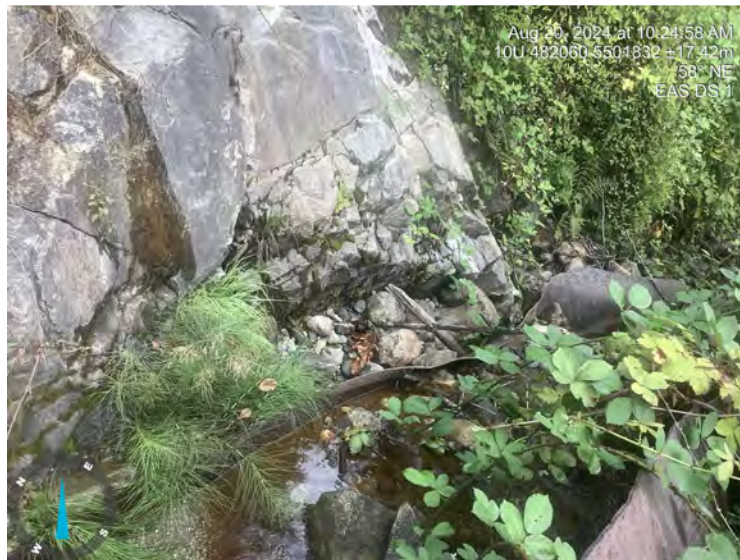
Photo: 3 Location: EAS DS 1 Description: DS view
