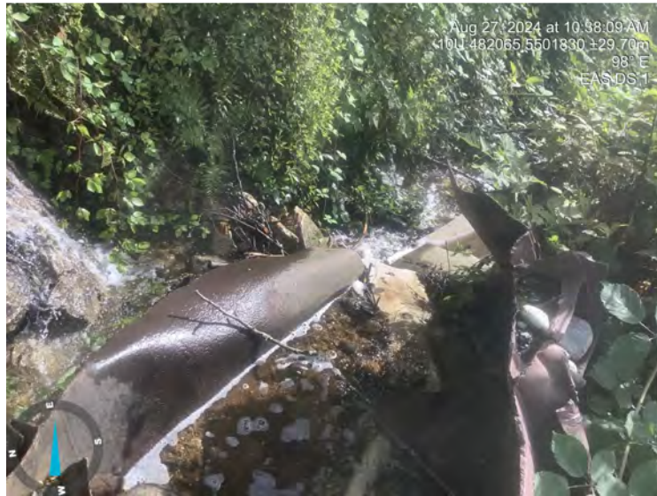
Photo: 3 Location: EAS DS 1 Description: DS view
