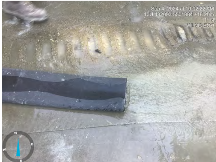
Photo: 2 Location: WLNG EOP Description: Across view
