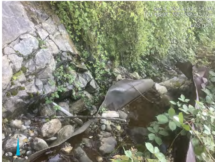
Photo: 3 Location: EAS DS 1 Description: DS view
