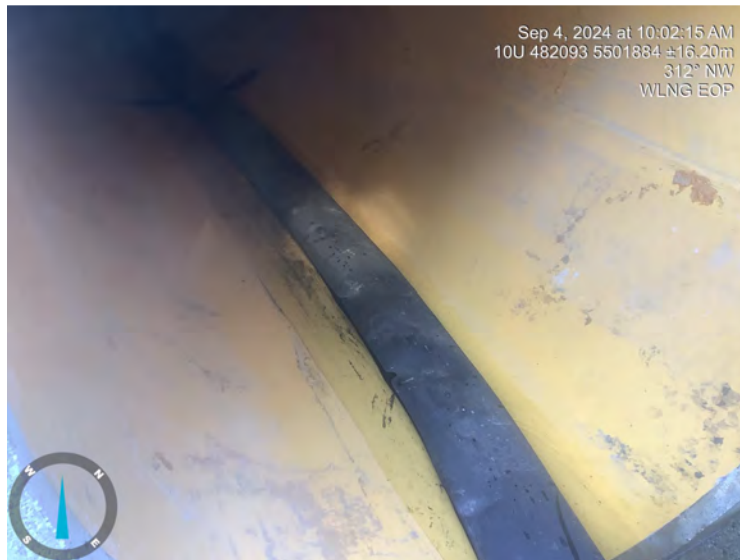
Photo: 1 Location: WLNG EOP Description: US view
