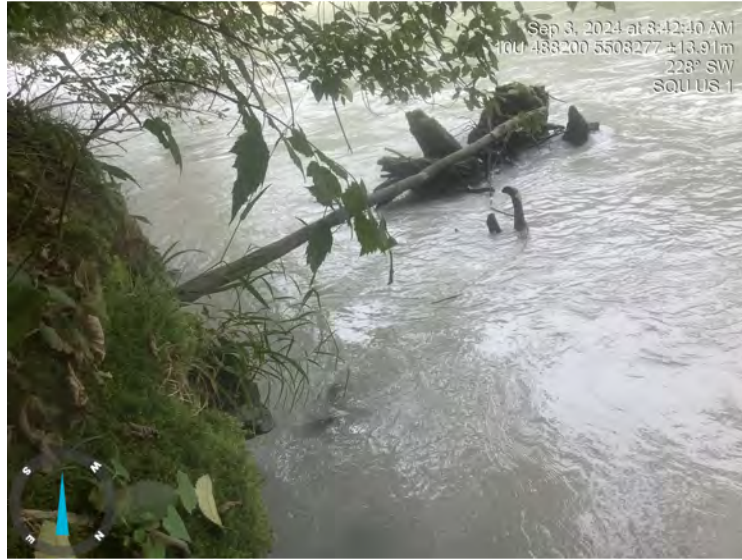
Photo: 3 Location: SQU US 1 Description: DS view
