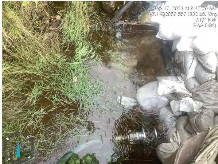
Photo: 2 Location: EAS DS 1 Description: Across view
