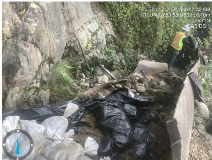
Photo: 3 Location: EAS DS 1 Description: DS view and isolated work area
