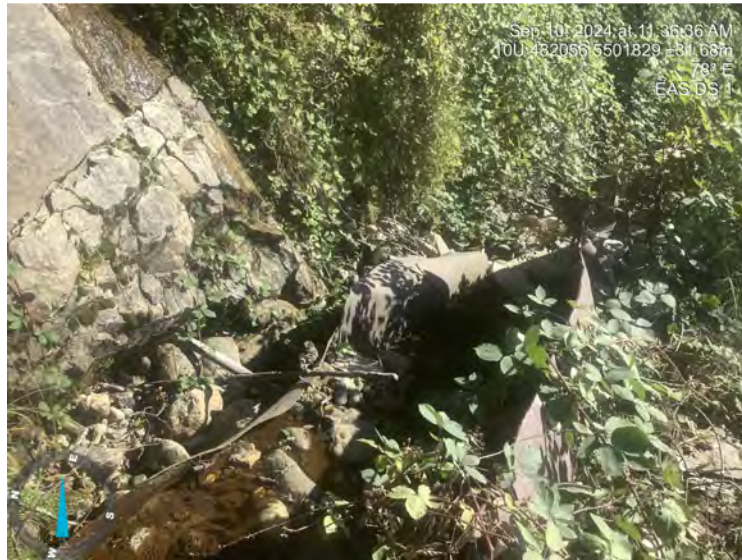
Photo: 3 Location: EAS DS 1 Description: DS view
