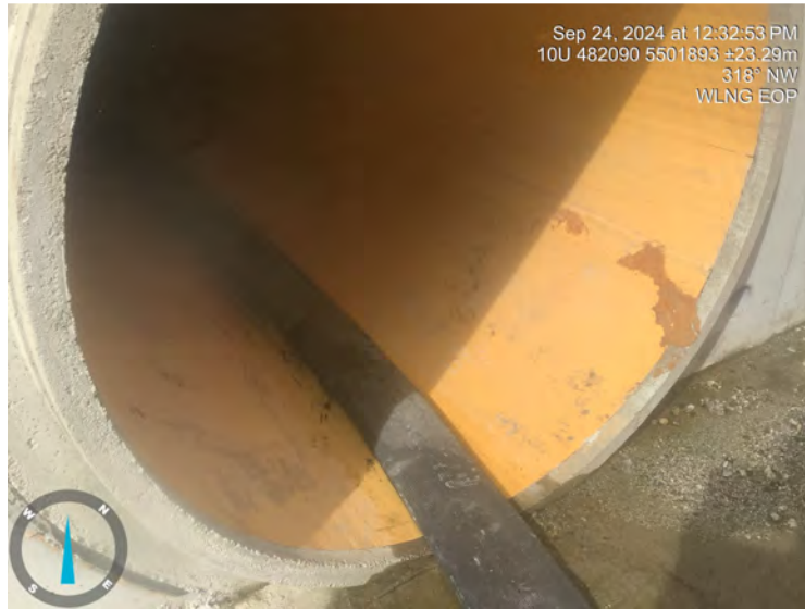
Photo: 1 Location: WLNG EOP Description: US view
