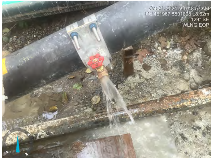
Photo: 2 Location: WLNG EOP Description: Discharge water from spigot.
