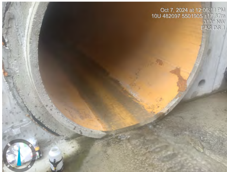
Photo: 1 Location: EAS DS 1 Description: US view
