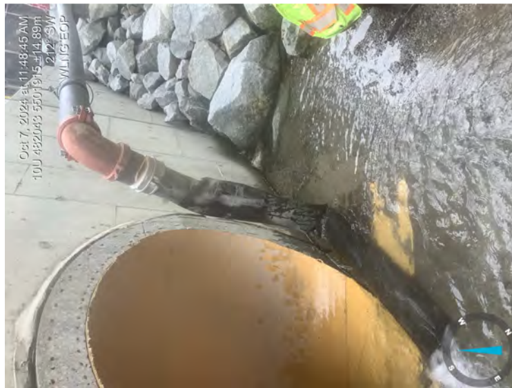
Photo: 1 Location: WLNG EOP Description: US view
