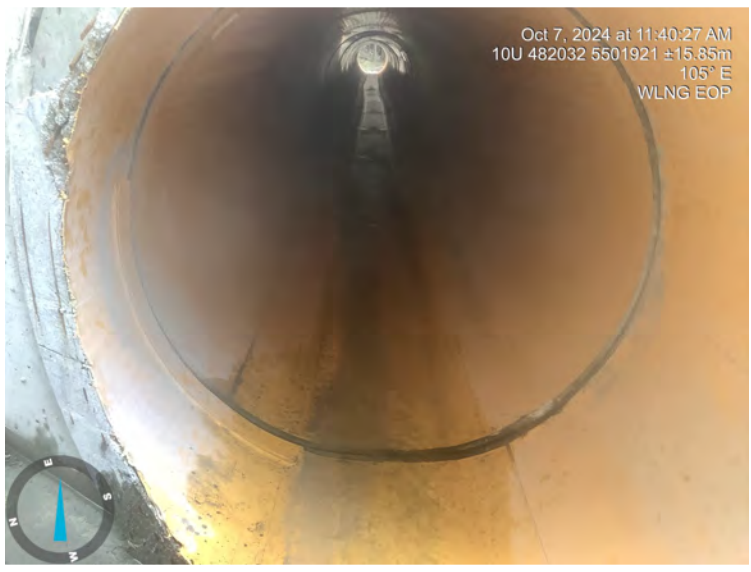
Photo: 3 Location: WLNQ EOP Description: DS view
