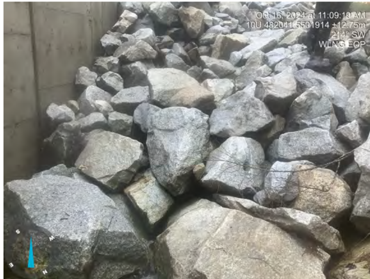
Photo: 1 Location: WLNG EOP Description: US view
