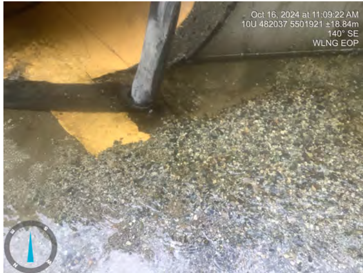
Photo: 2 Location: WLNG EOP Description: Across view
