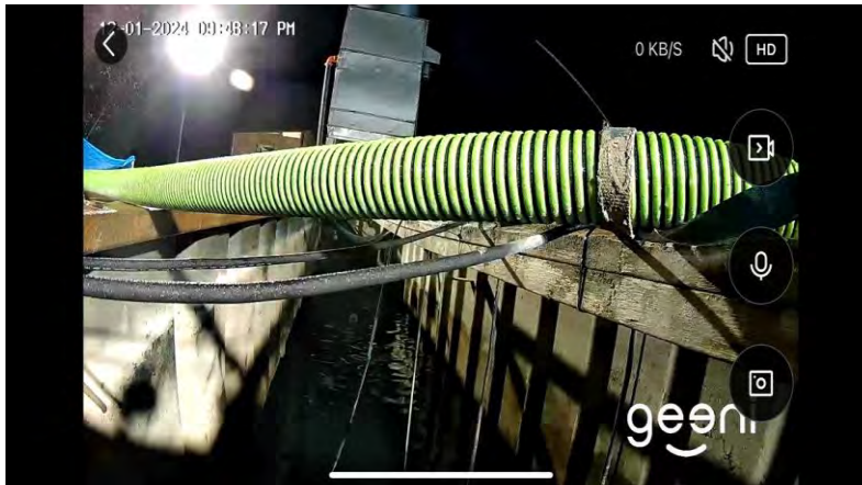
Photo 7: No visible sheen observed in the WTP water, December 1 st
