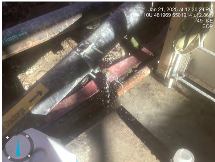
Photo: 1 Location: EOP Description: Sampling location
