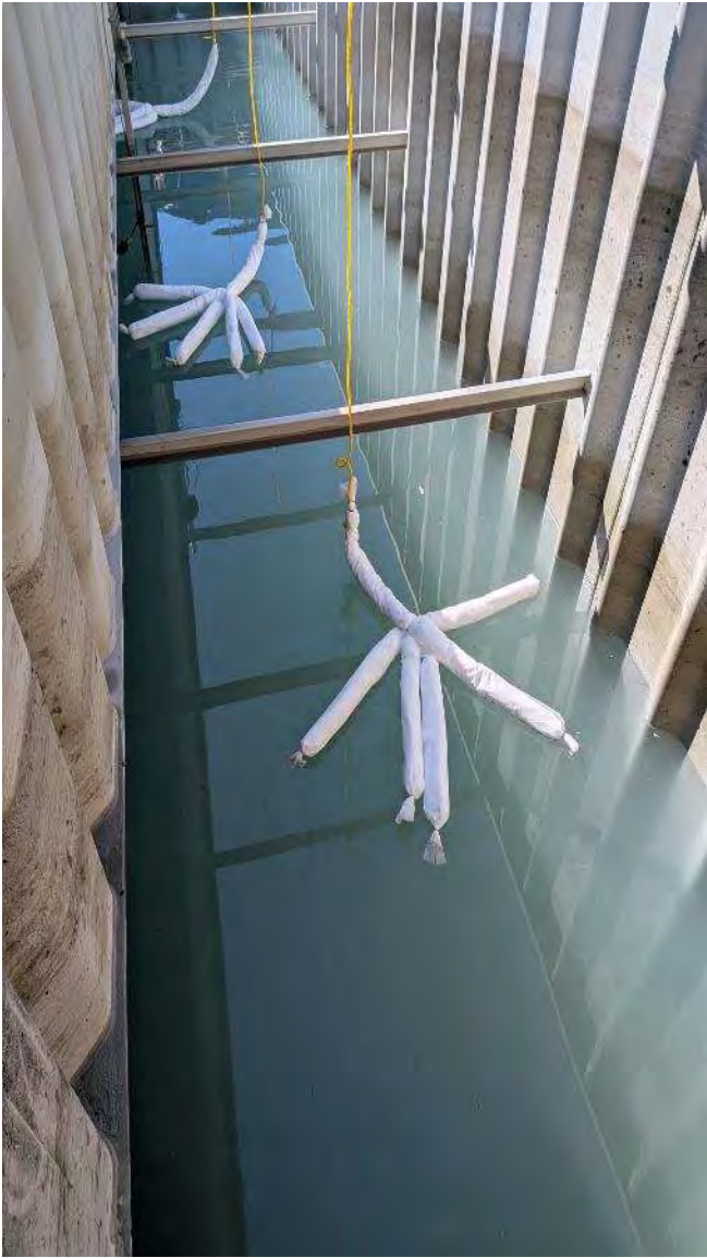
Photo 5: No visible sheen observed in the CP2 WTP water, April 29. Spill booms installed as a precaution.
