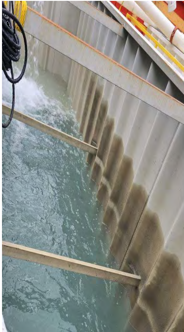
Photo 2: No visible sheen observed in the CP2 WTP, May 25
